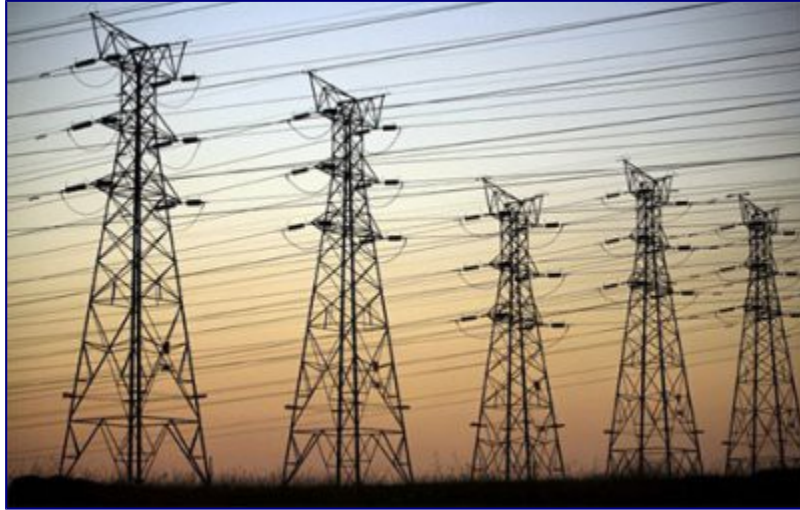
Power lines will be history.
