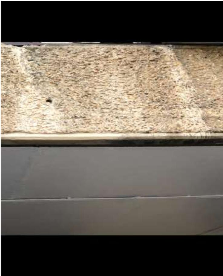
The lower lighter area on the left of the photo is our repair area. The area on the right is where the rainwater has cleaned the concrete. This shows the comparison in colours and shows how close the repair matches a clean area of concrete. The repair area is quite fresh and the brightness will dull down slightly and the exposed stones will lose the residue on them over the coming winter months to be more prominent within the repair.
