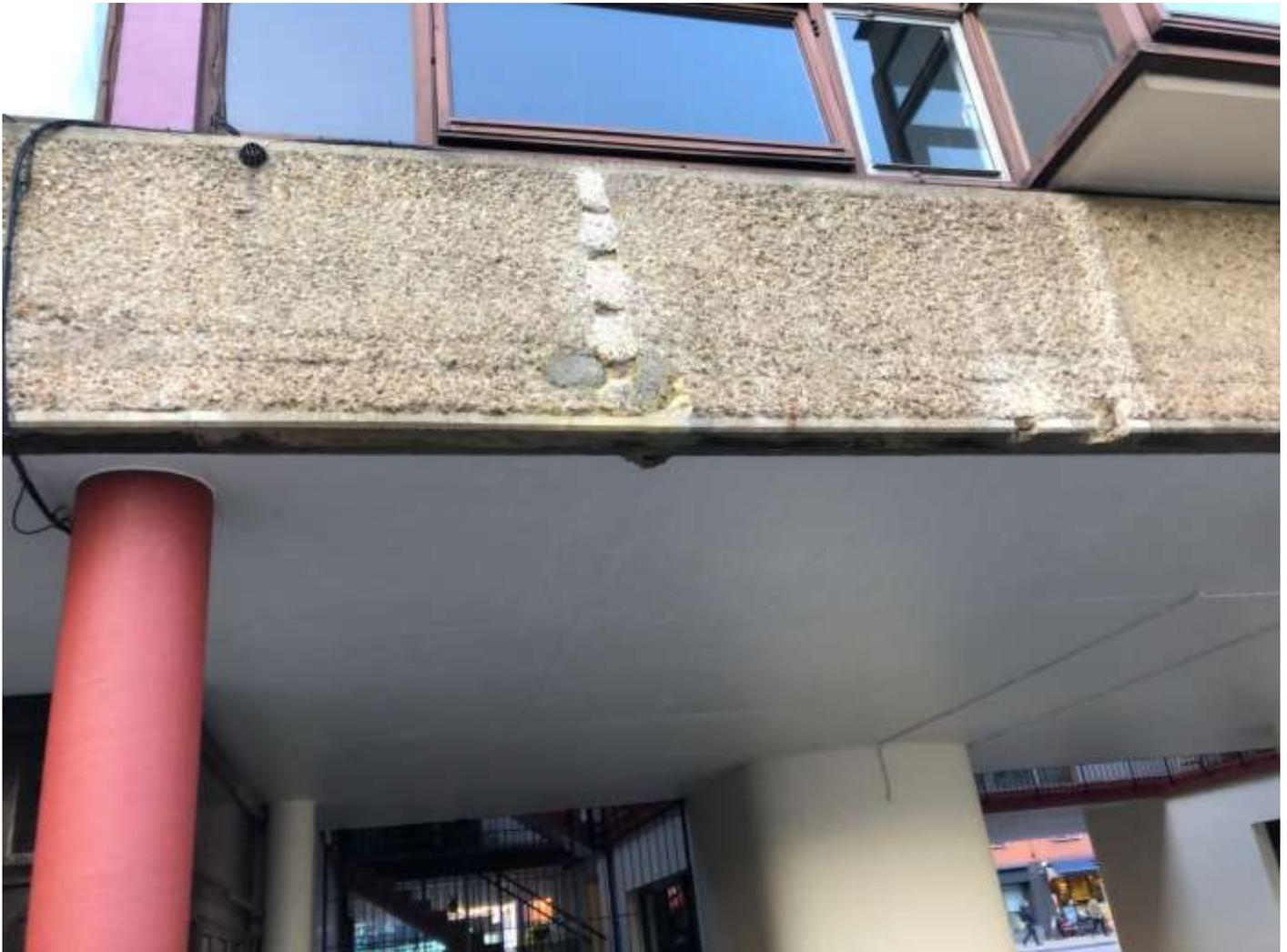
This photo shows some of the various samples mixed and applied in the quest for a 'best match'. The top uppermost samples applied are exactly as the concrete that was poured when the building was first constructed but we must take into account how the colour has changed over time and how it looks right now.
