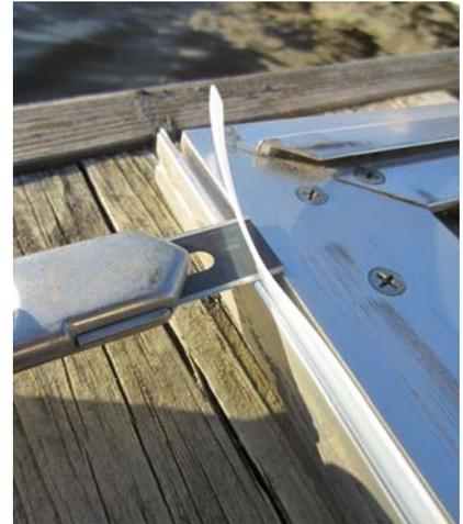
**A picture showing how I used the carpet cutter to trim the “top” of the Slick Strip off.**
