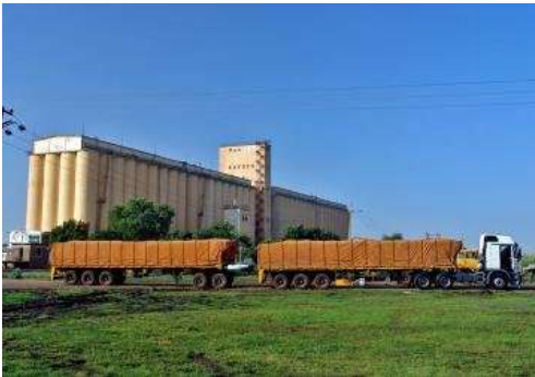
Gadarif silo the biggest In Sudan
